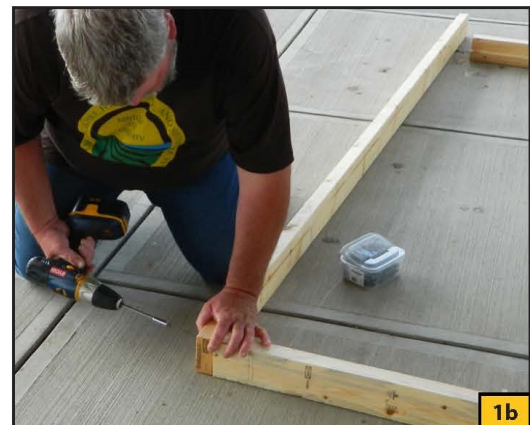
A couple of deck screws per corner secure the base assembly 2x4s.
