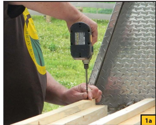
Drywall screws are used to attach the cleats.
